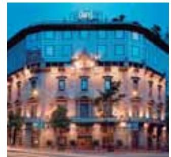
Hotel refurbishment. Hotel Claris 5 * Barcelona, Spain. ECOi
